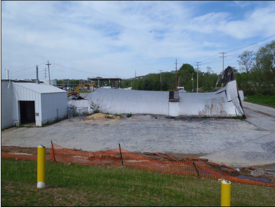
Photo 1: Building 51 (view looking west) during initial demolition (May 2011).
