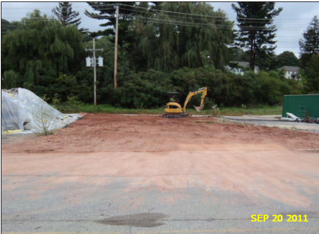
Photo 4: View looking north at backfilled excavation of former Building 51 area.
