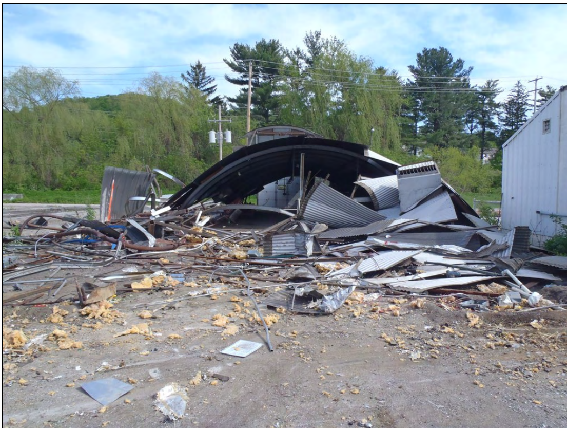
Photo 2: View looking north of demolition of former Building 51 (May 2011).
